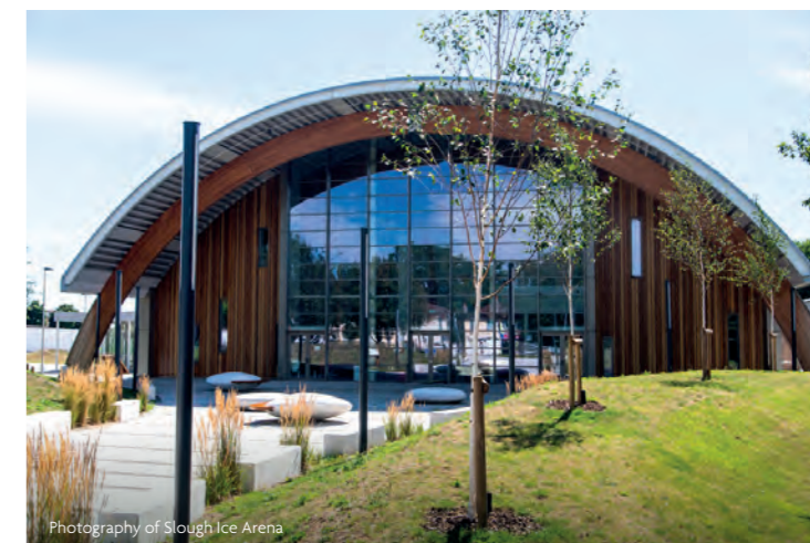
Photography of Slough Ice Arena
